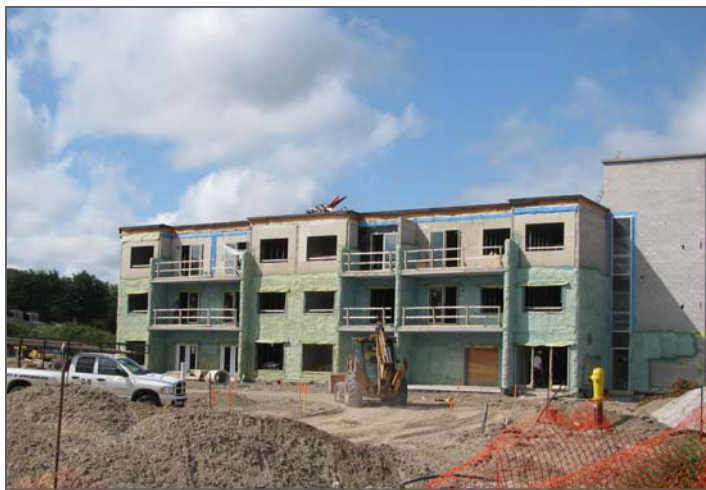
Above: Construction continues on the addition
